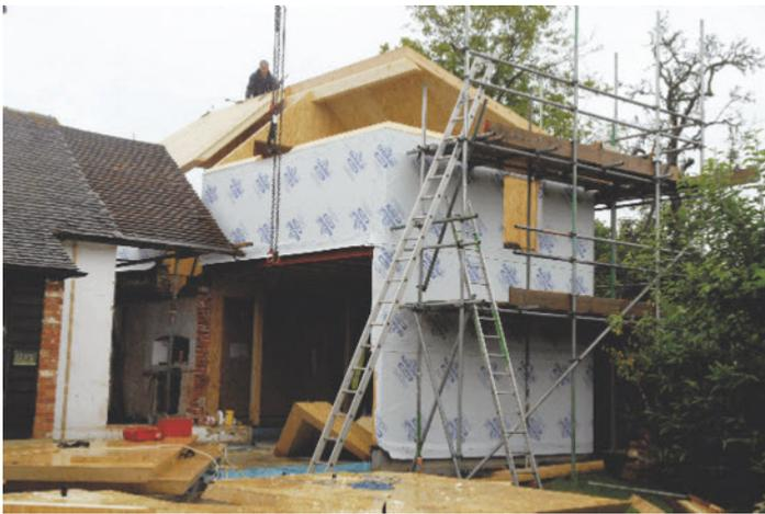
When combined with an MVHR system, this construction method is one of the most effective ways of creating an energy efficient building, and can significantly reduce heating and cooling requirements.
